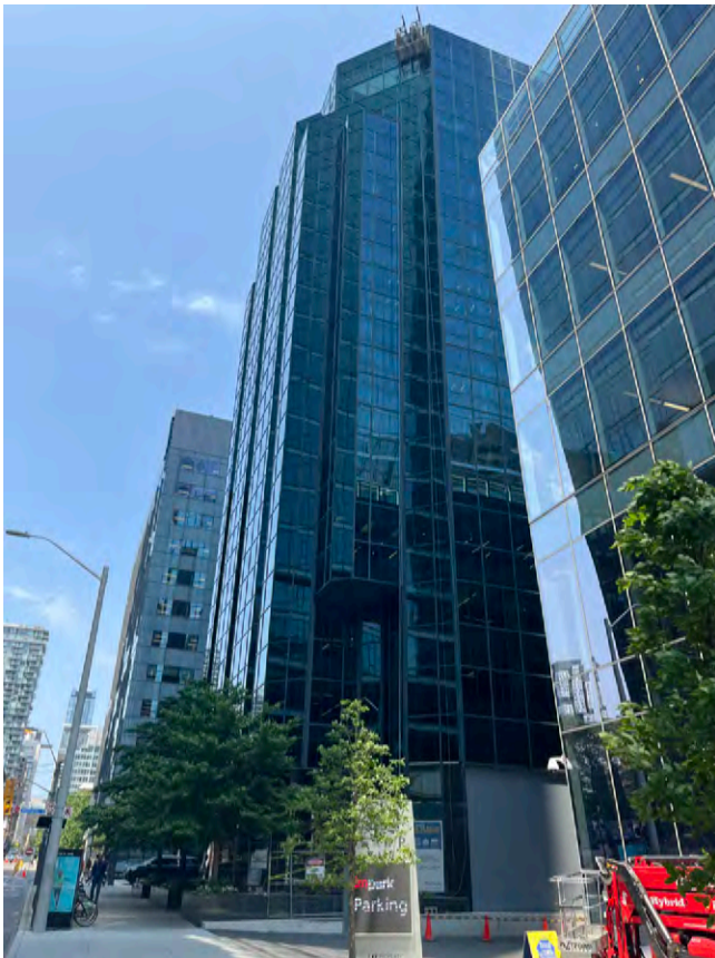
6. South and partial west elevation of 145 Wellington Street West (background), and 160 Front Street West (foreground) (Source: ERA Architects).
